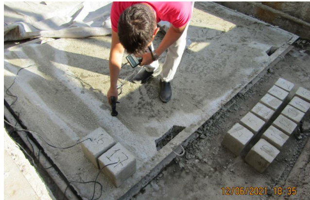
Figure 2 – Operational control of the strength of large samples (road slab) by ultrasound method
