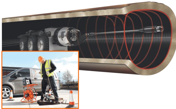
Figure 4 – Example of using lasers to monitor the internal condition of pipes
