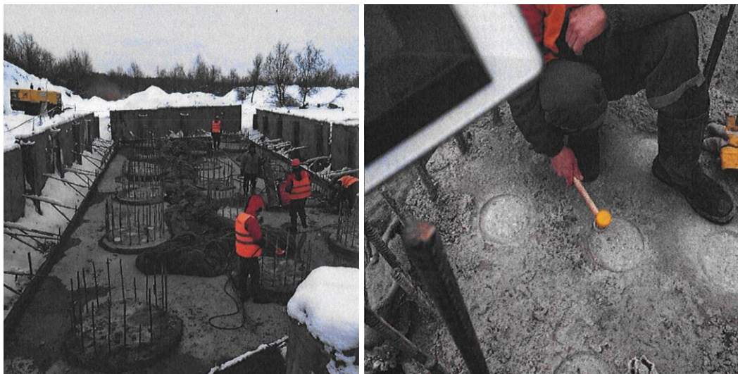
Figure 1 – Construction site of 18 bored piles
