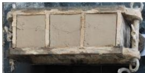
b) Micro-cracks appearing on the surface of the specimen
