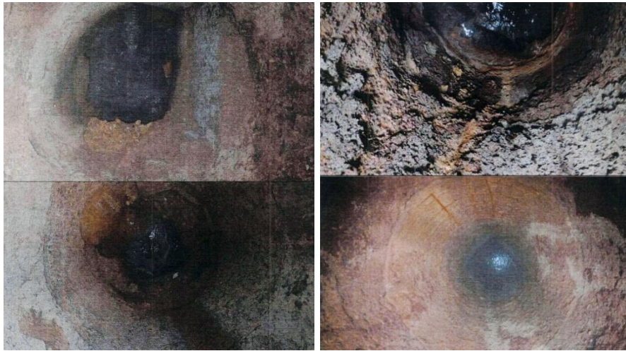
Figure 2 – Pipelines condition before CIPP installation
