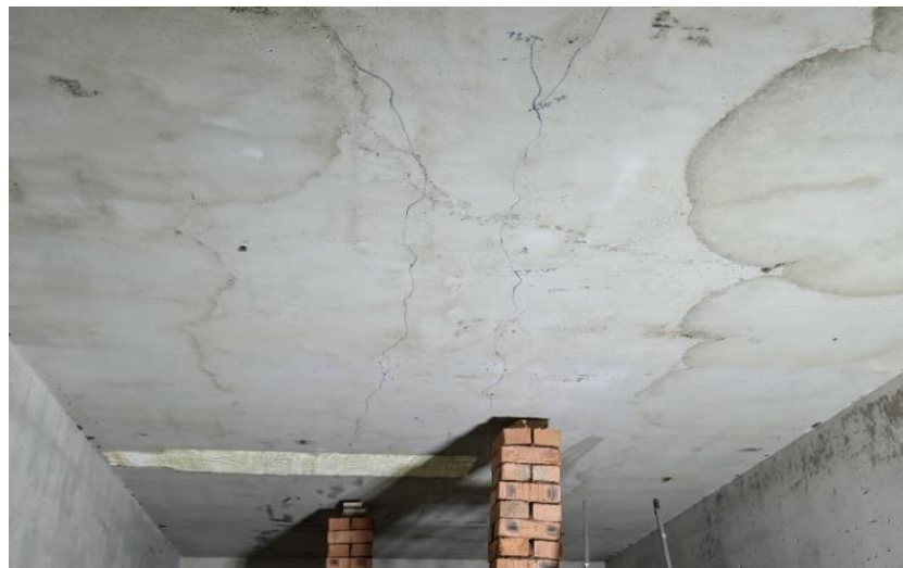
Figure 12 – Cracks in the ceiling slab
