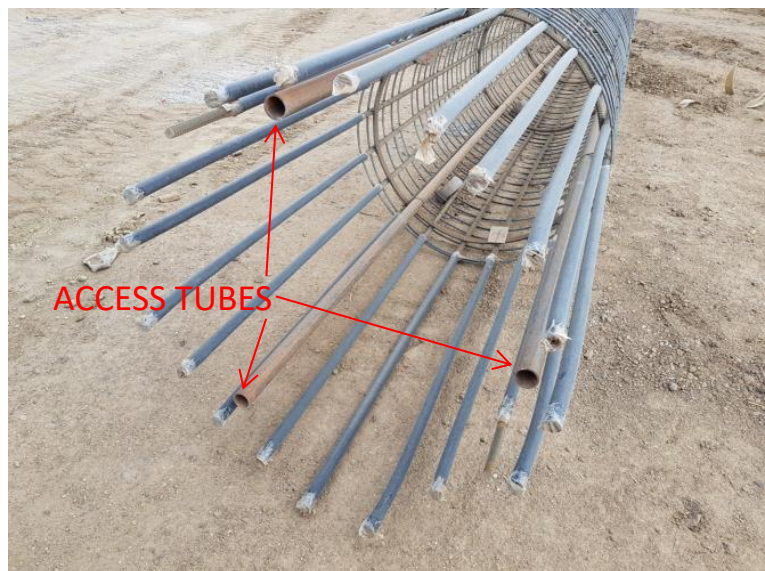
Figure 3 – Typical access tube configurations: a) scanning along three measurement directions; b) scanning along the perimeter and diagonals (six measurement directions).
