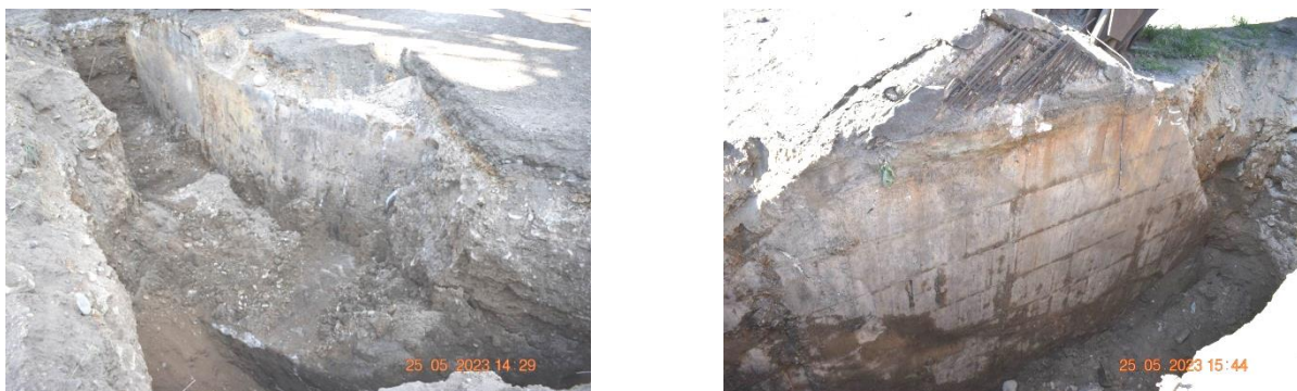
Figure 2 – General view of the opened test pits
