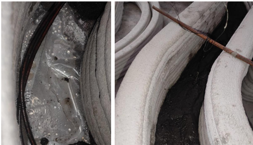
Figure 4 – Reinforcing and pouring the voids with heavy concrete
