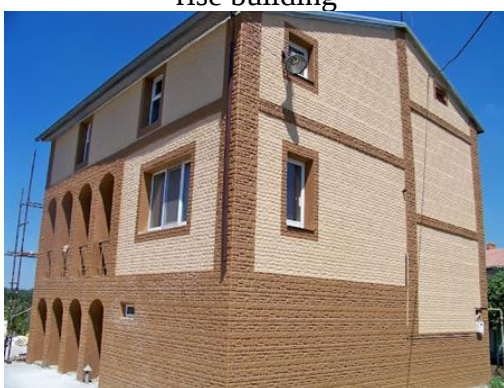
c) Wall made of a thermal panel
