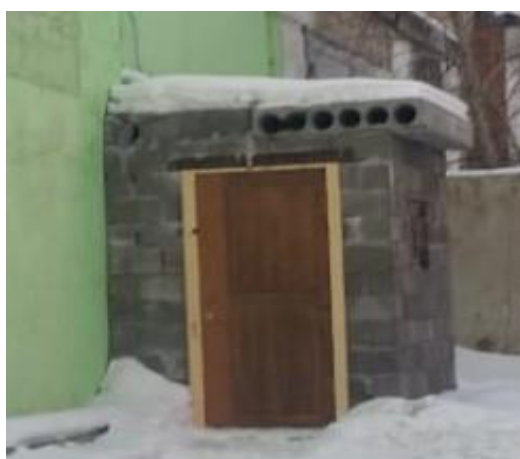
Figure 10 – Full-scale tests of the manufactured pilot-industrial batch of products «Hollow wall stone with ash-and-slag waste» in the form of construction of an extension to the production workshop of EcostroyNII-PV LLP
