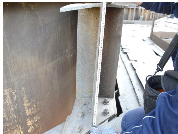
Figure 9 – Rolls and loss of local stability of the walls of the support beams of gas outlet shafts characteristic for beams at the site level at level +49.200
