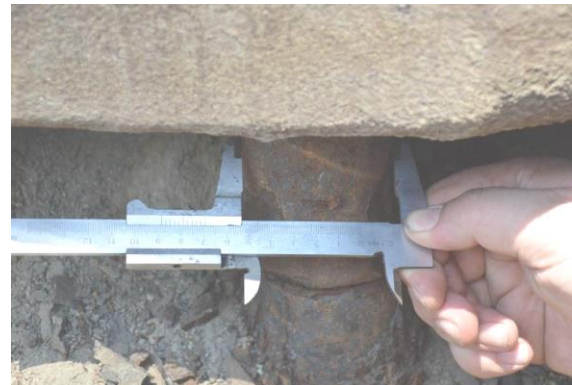
Figure 4 – Continuous irregular corrosion of foundation bolts
