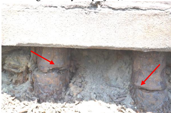
Figure 3 – Breakage of foundation bolts
