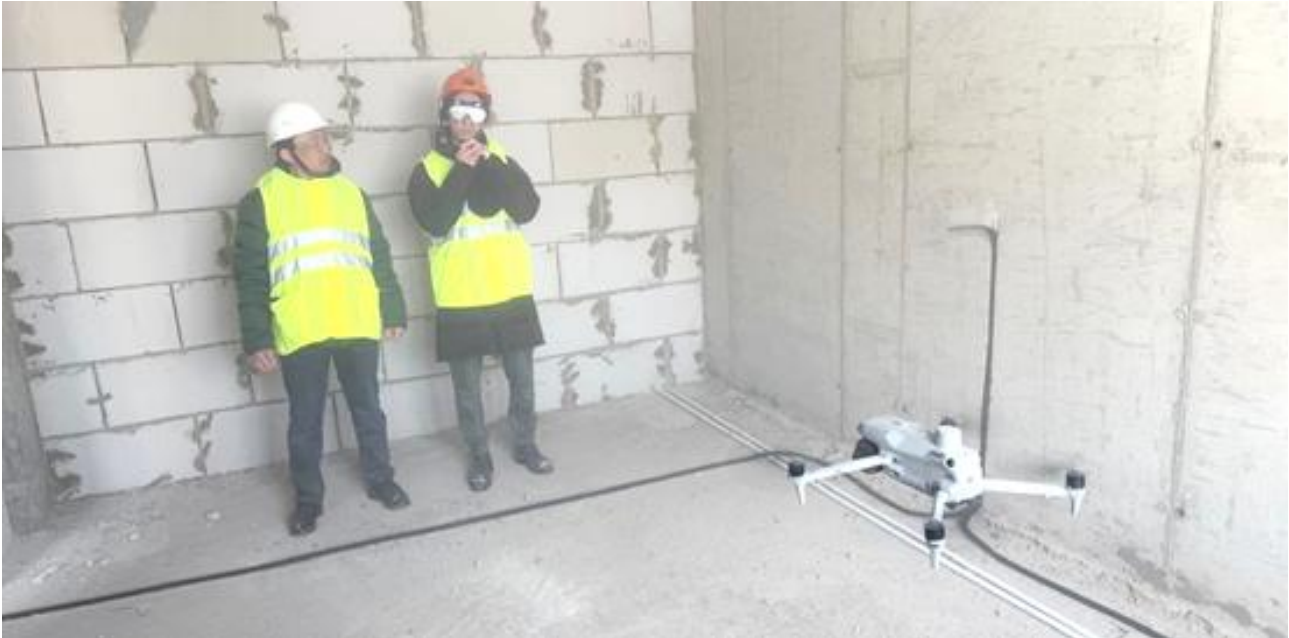
Figure 3 – DJI Matrice 4E UAV and construction site workers before an experimental video recording session inside a building under construction
