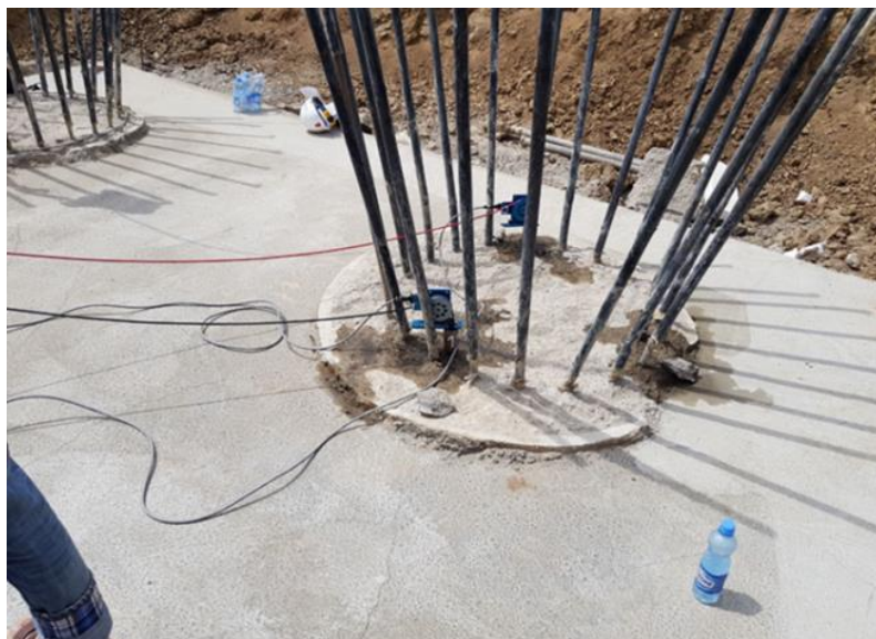
Figure 5 – CSL pile testing with two probes
