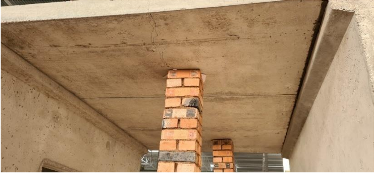
Figure 9 – View of safety supports under the interblock corridor slab
