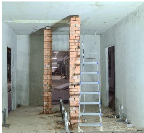
Figure 4 – Deflection gauges and safety supports under the ceiling slab
