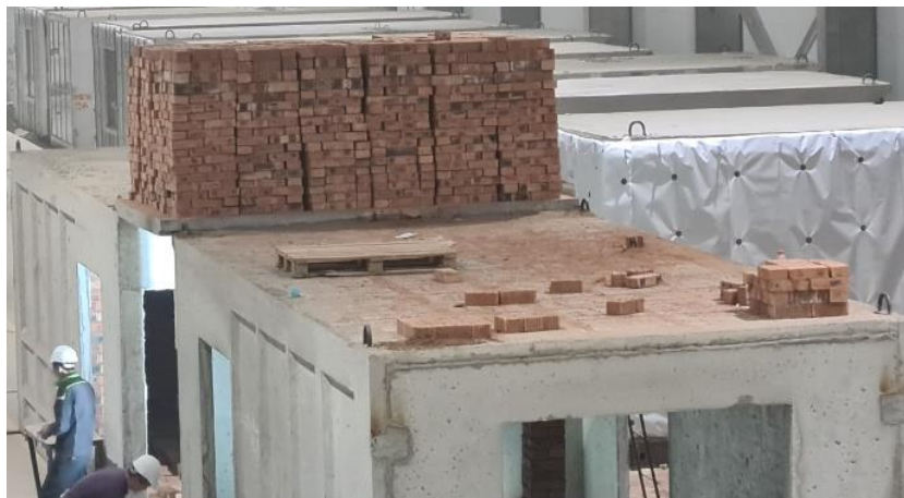
Figure 7 – View of interlocking floor slab loaded with brick
